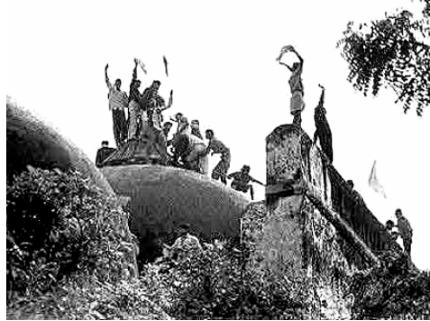
Demolition of Babri Masjid
